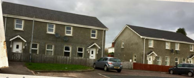
New Social Housing at Glenavy Gardens
